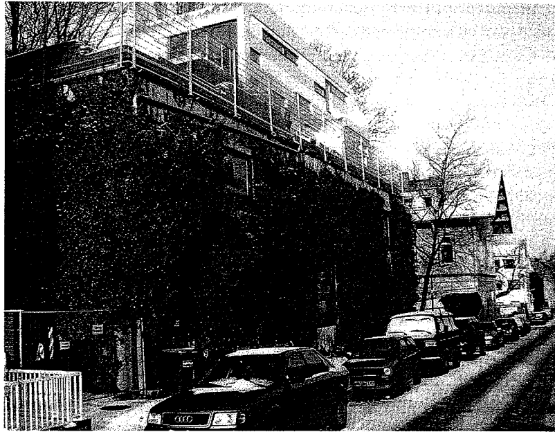
Fig. 7. Former air-raid shelter in the Berliner Strasse, Bremen, current condition. The shelter is hidden behind plants and has functionless windows. There is a residence on top. (Photo: Marc Buggeln.)
